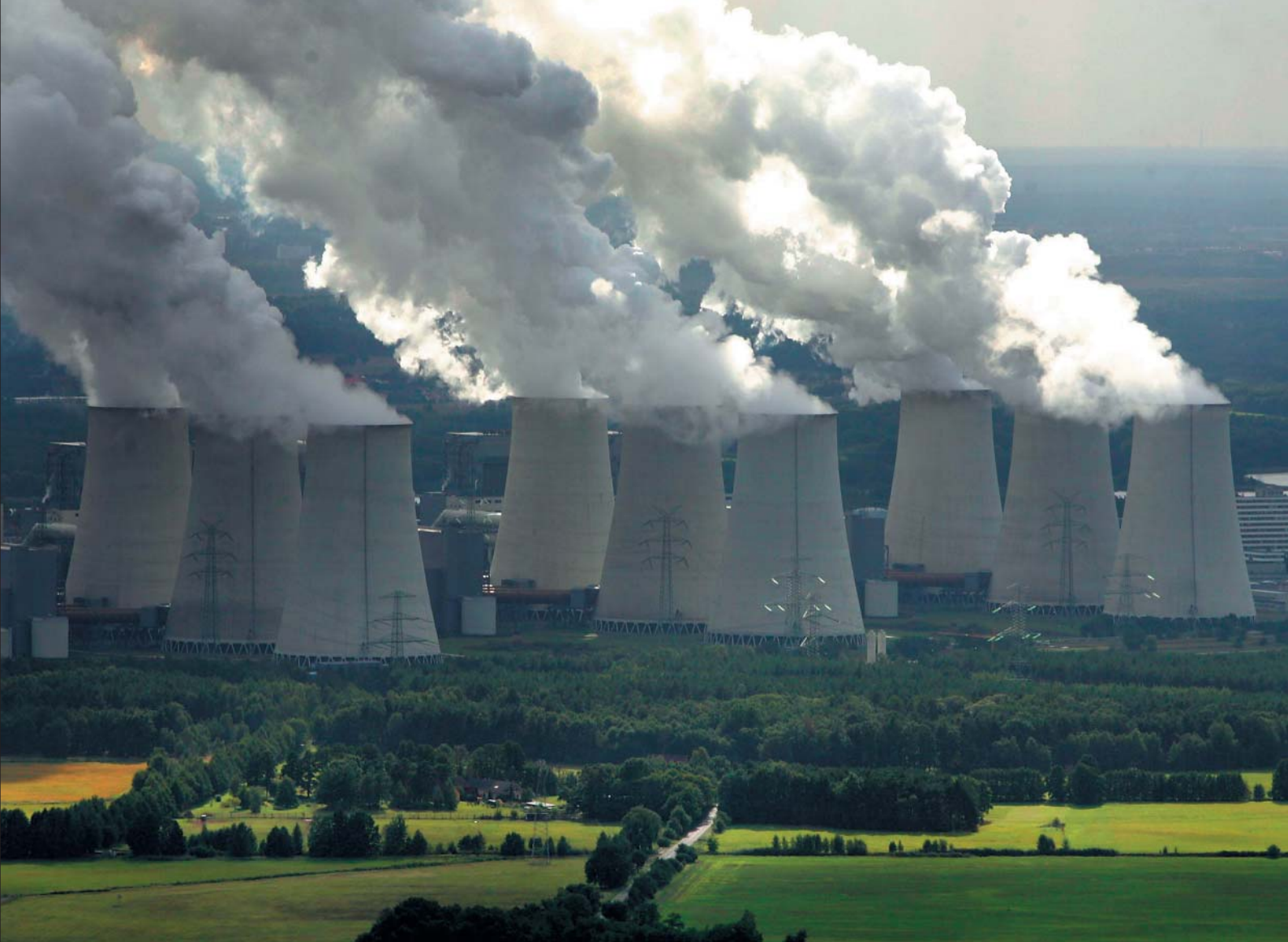
Cooling towers by a power plant.
